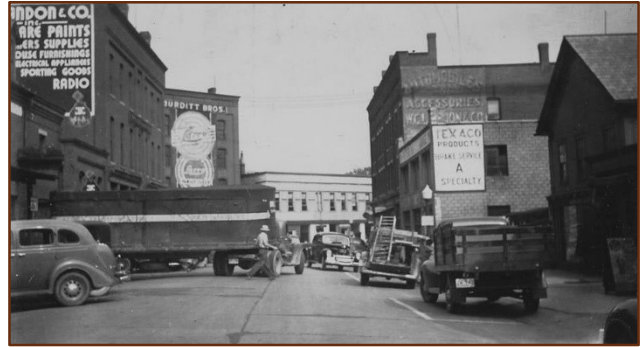
Evelyn Street and Freight Corner before demolition in the late-1960s
